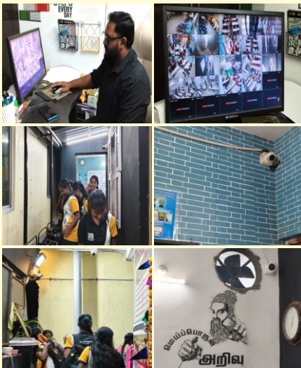
19. CCTV Camera Facility
